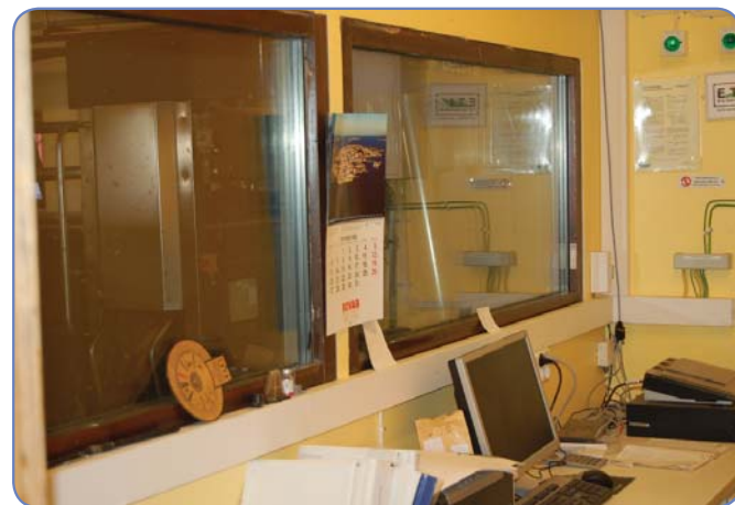
From the office there is an overview of the VMS units.
